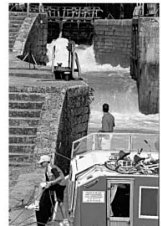
Triple staircase lock at Laurens. Note how the Midi staircases are worked with intermediate gates open, so that water cascades impressively into the lower chamber. Miss. Alain Felix
